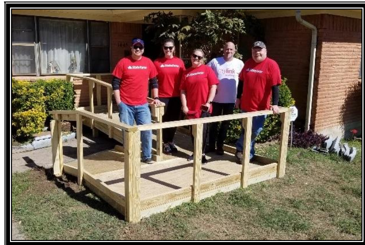
State Farm Employees celebrate two of the five completed ramps.
